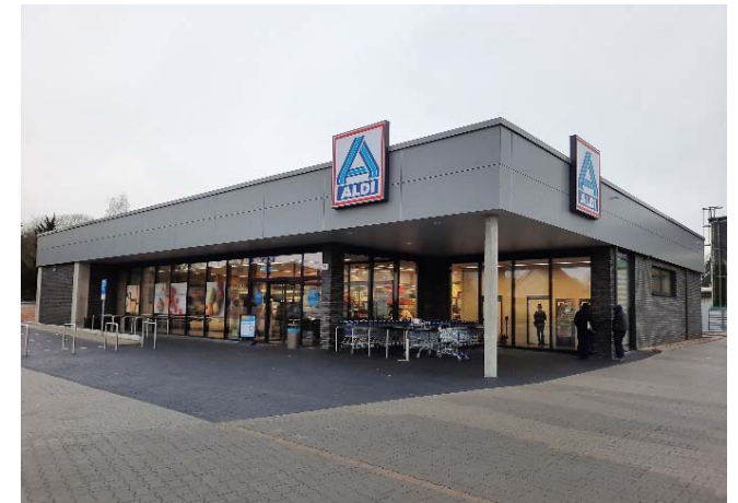
... looks like newly built after the refurbishment.
