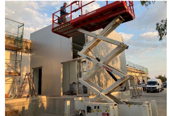
Supply ramp for EDEKA
