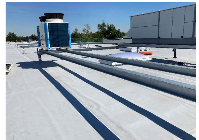
Renewed roof with technical facilities built upon
