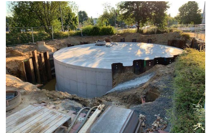
New sprinklertank
